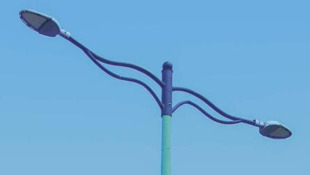
**Advantages of GRP poles:** These are high corrosion resistance poles and are safe in accidents. These poles are light in weight and fast and easy for installation. GRP poles are electrically non conductive.
